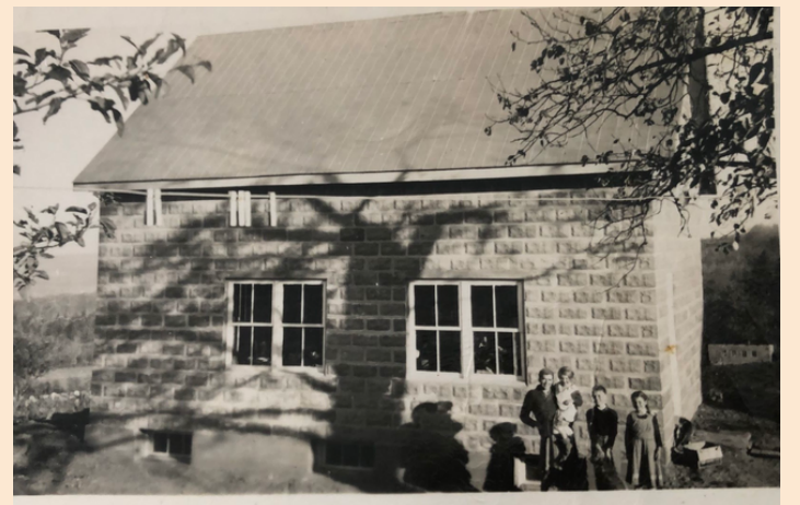
The new house - after the fire
